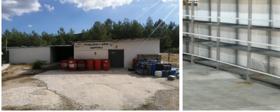
Figure 12: Hazardous Waste Warehouse
